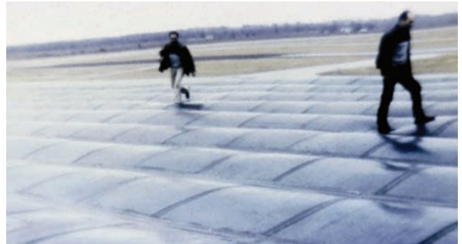
Photo 2: Fluttering membrane. No air barrier at deck leads to an idea for a Disney World ride.
